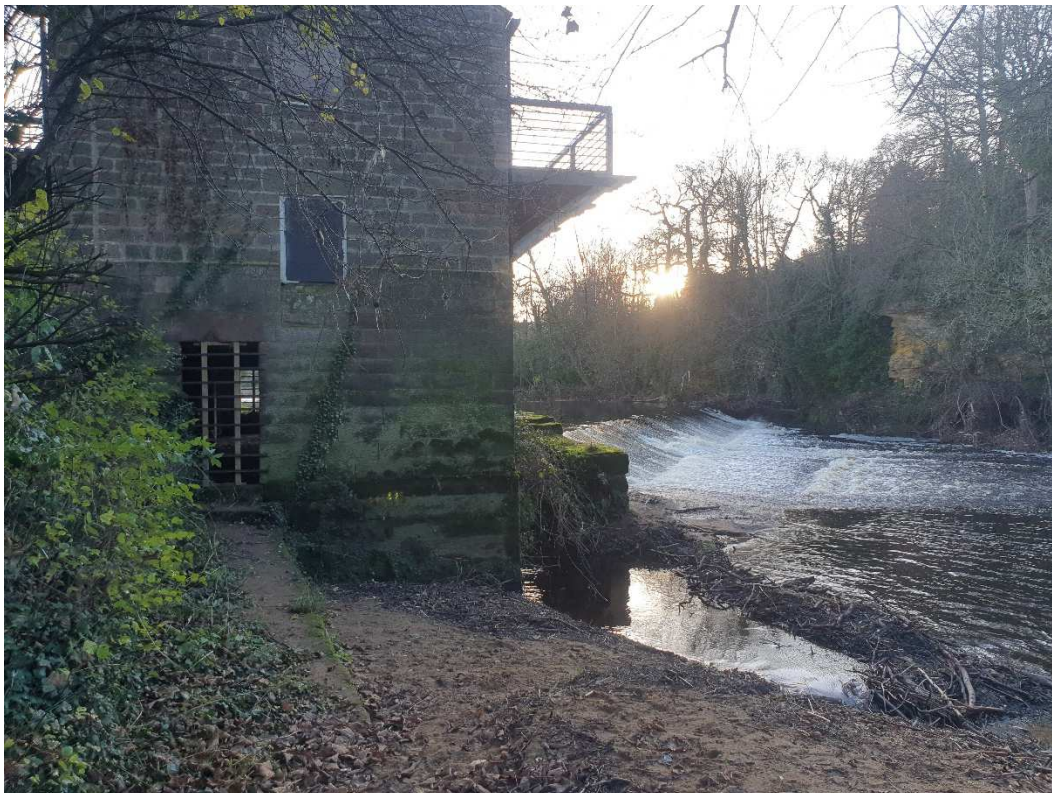
Figure 9: Silted area downstream – proposed site of turbine installation
