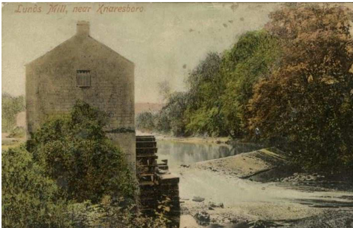
Figure 1: The mill and weir prior to 1909
