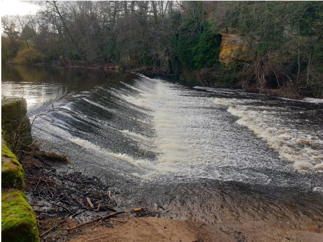
Figure 4: Weir, return view upstream from mill wheelpit wall
