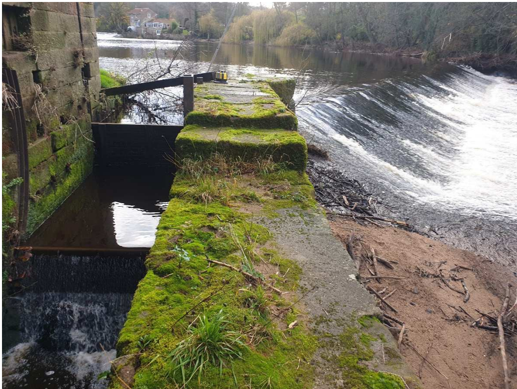
Figure 7: Wheelpit, outer wall, and weir, looking upstream
