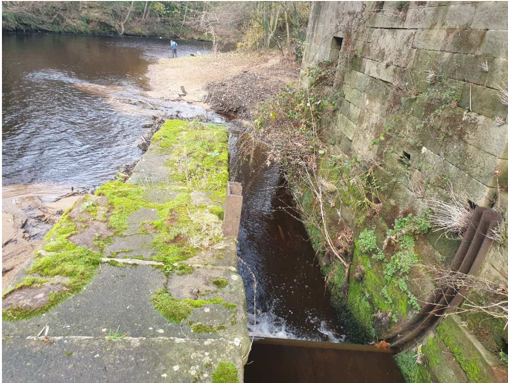
Figure 6: Wheelpit, walls, and iron guides, looking downstream
