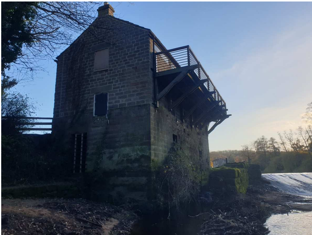
Figure 5: Mill, wheelpit, outer wall, weir - view upstream
