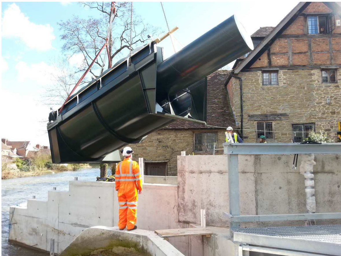
Figure 11: Installing a 30kW screw in an open compact trough
